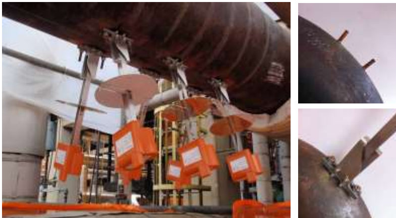
Permasense WT100/WT210 sensor, attached with stud-welded bolts (courtesy Permasense)
